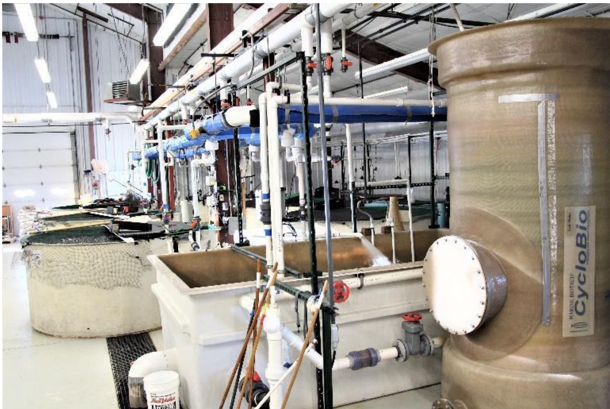
Figure 8. An Indoor Recirculating Aquaculture System
