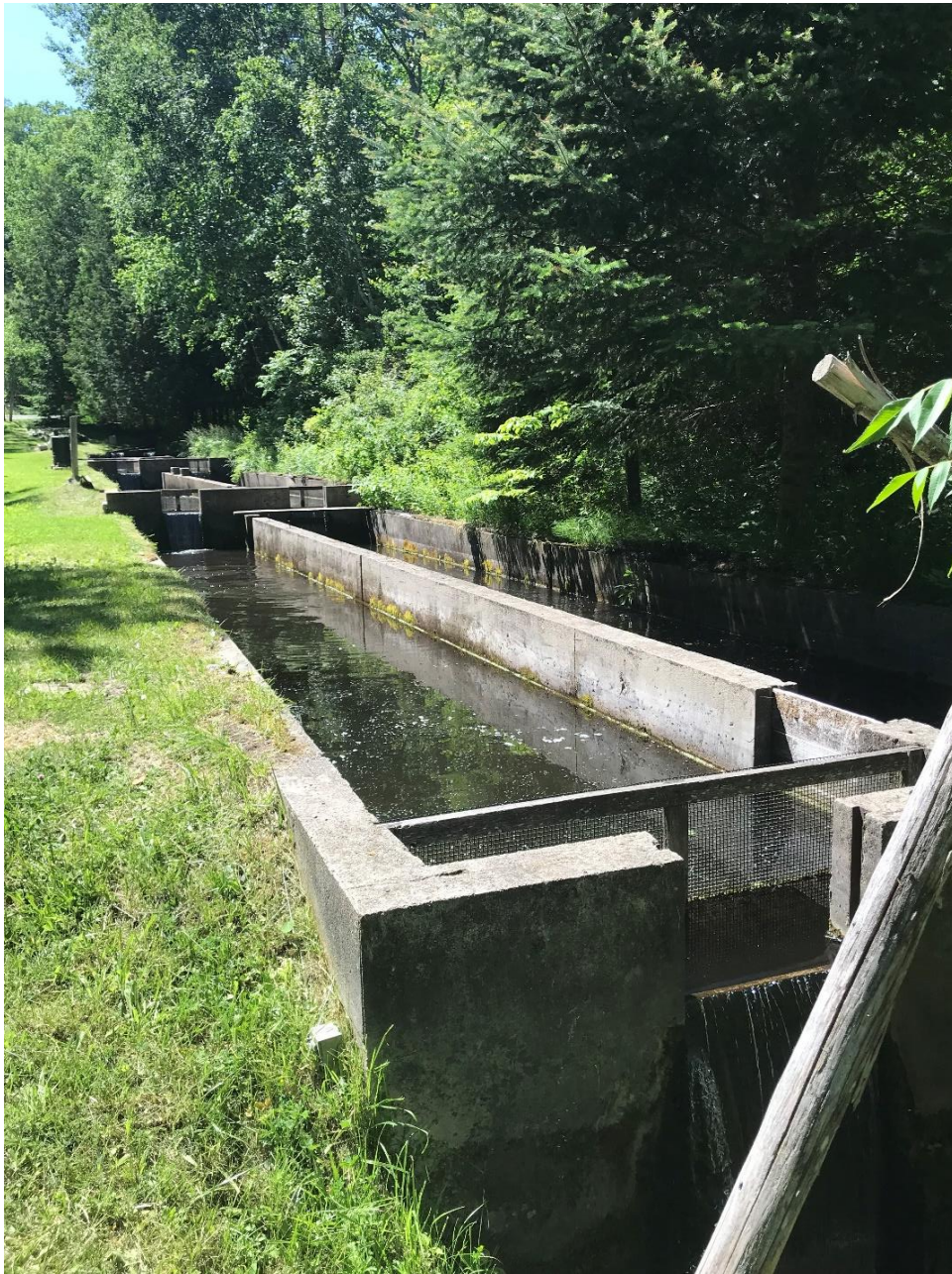
Figure 7. Concrete Single Pass Raceways with Brown Trout at a Michigan Trout Farm
